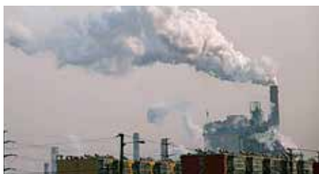
Steel plant, Hebei Province (Irish Times, 18/04/14)
